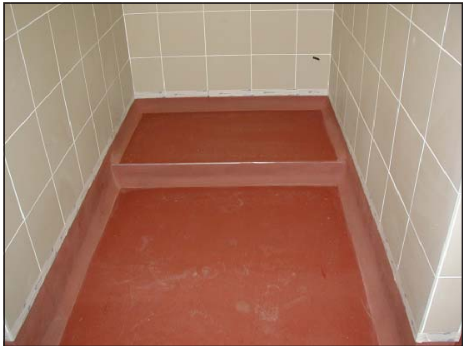
A touchstone Resin floor in the kennels of the British Transport Police's Dog Training School
