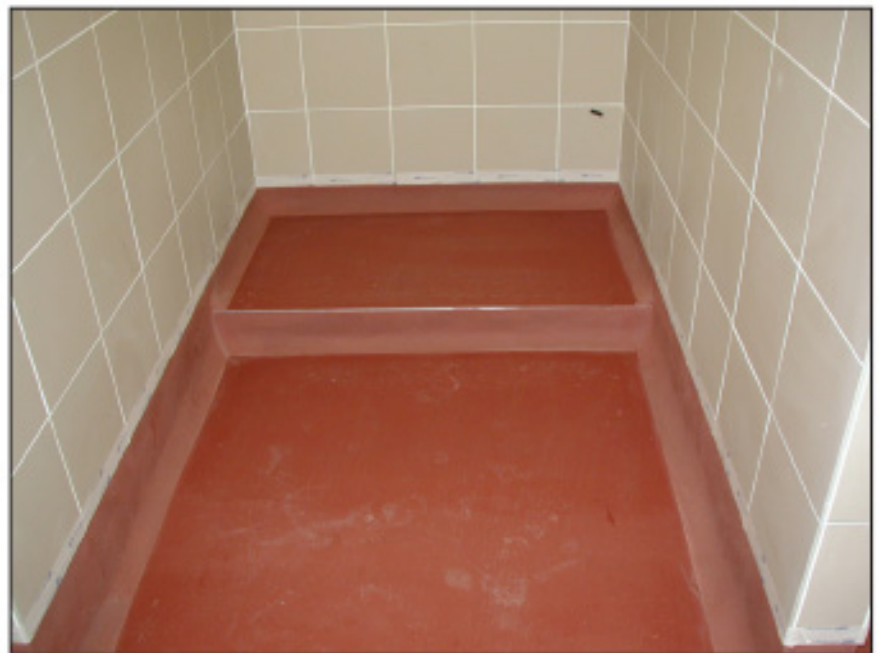
A touchstone Resin floor in the kennels of the British Transport Police's Dog Training School
